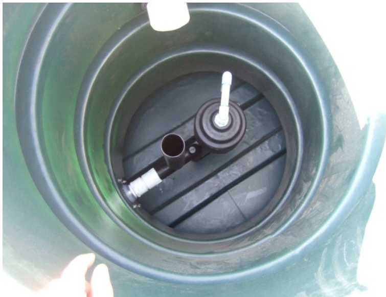
Figure 6. Dosing siphon - internal view
