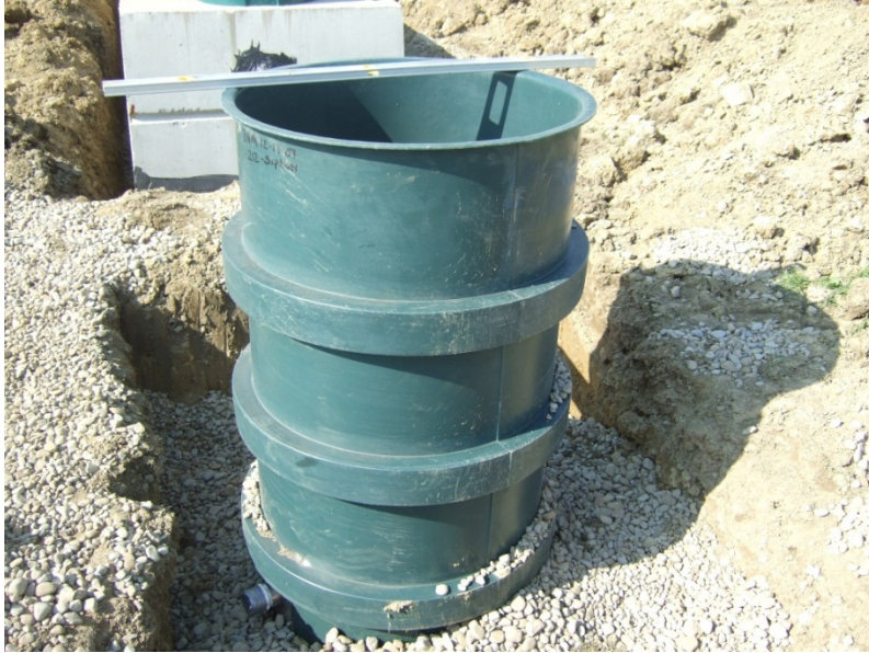
Figure 5. Dosing siphon - external view
